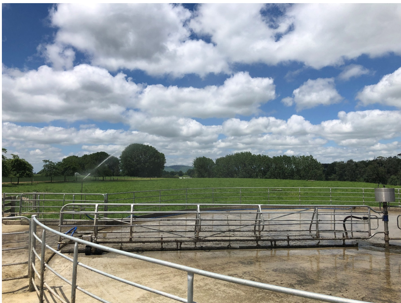
FIGURE 5: SPRINKLER AT BACK OF YARD
