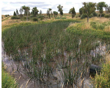
Constructed wetlands are typically planted with native plant species.
