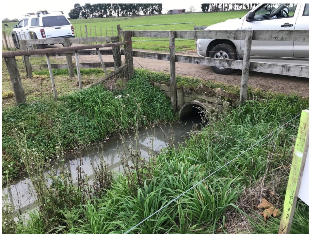
Plate 19: Management Unit 9a, culvert. 2 June 2021.
